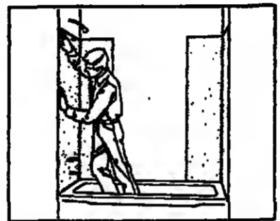
Side panels are installed first. Each of these folds around onto back wall so rear panel fits on top.
